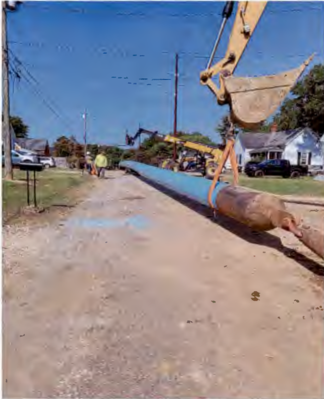
24-inch Water Transmission Line project pictures.
