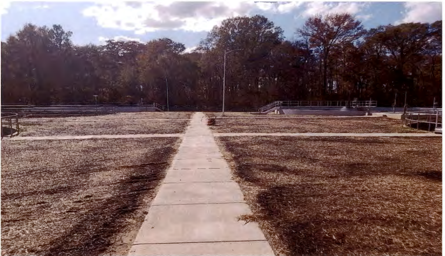
Construction upgrade seeded with grass.
