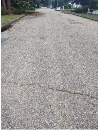
Figures 5 & 6: Transverse Cracking and Block Cracking as seen on Orange Avenue and W. Pearsall Street
