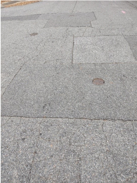
Figures 9 & 10: Utility patches can affect ride quality. Tree roots buckling pavement on W. Godwin Street creating an uneven, rough riding surface.
