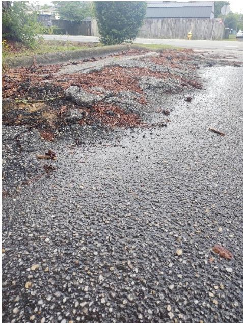
Figures 9 & 10: Utility patches can affect ride quality. Tree roots buckling pavement on W. Godwin Street creating an uneven, rough riding surface.
