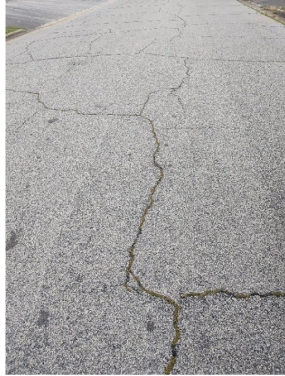
Figures 5 & 6: Transverse Cracking and Block Cracking as seen on Orange Avenue and W. Pearsall Street
