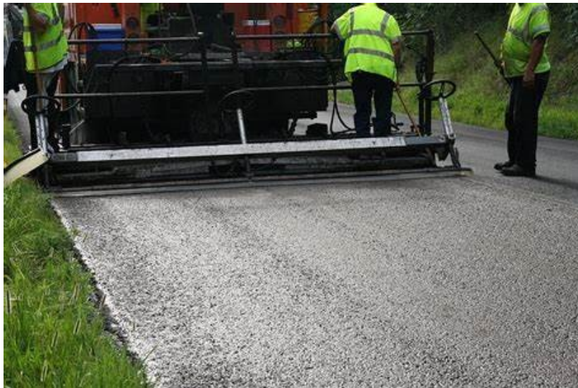
Figure 18: Typical Microsurfacing for preservation of roads
